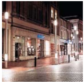
Fig. 6.41 Combined lighting units with high mount lanterns and bollard height lighting
