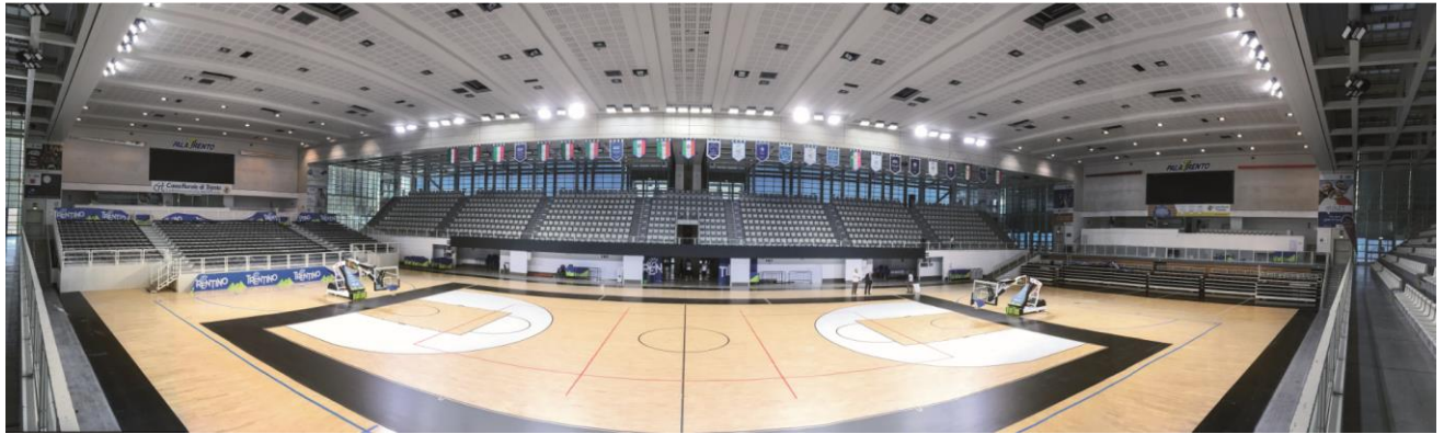
Image 2: A total of 92 symmetrical and asymmetrical floodlights can achieve lighting levels of up to 3400 lux
