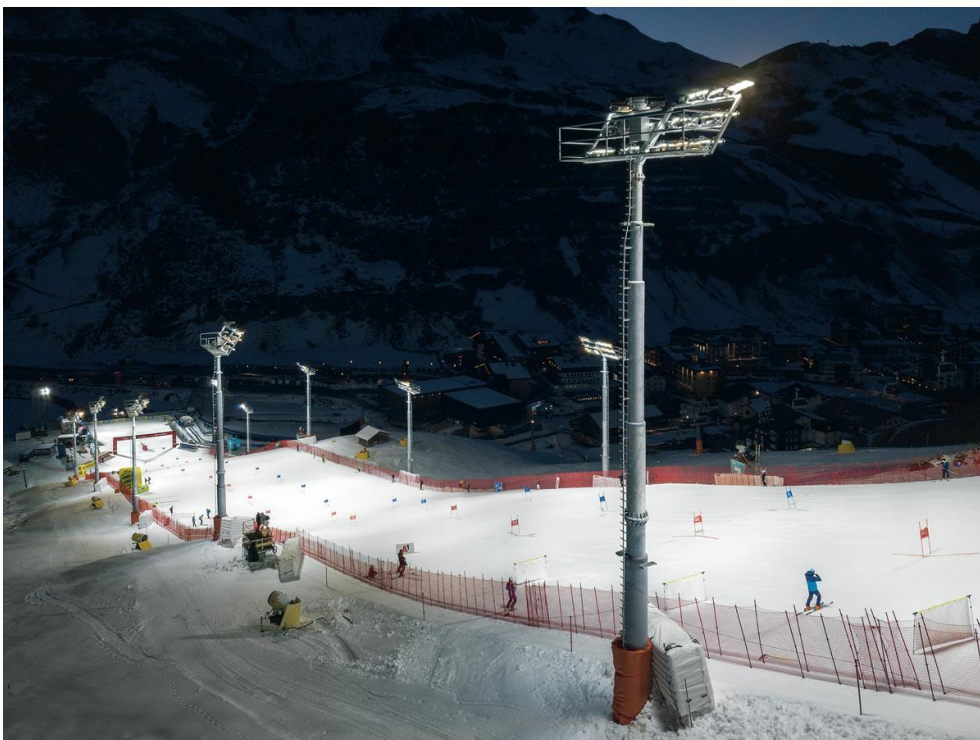
State-of-the-art floodlighting system for the Flexenarena in Zürs
