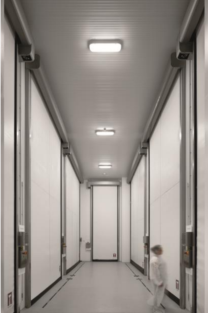
Image 2: The latest LED technology enables ForceLED to guarantee excellent energy efficiency and longer maintenance intervals in the storage facilities.
