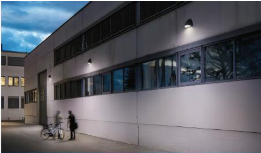
Image 1: The directional LED light source of Piazza II ensures light is directed only where it is required
