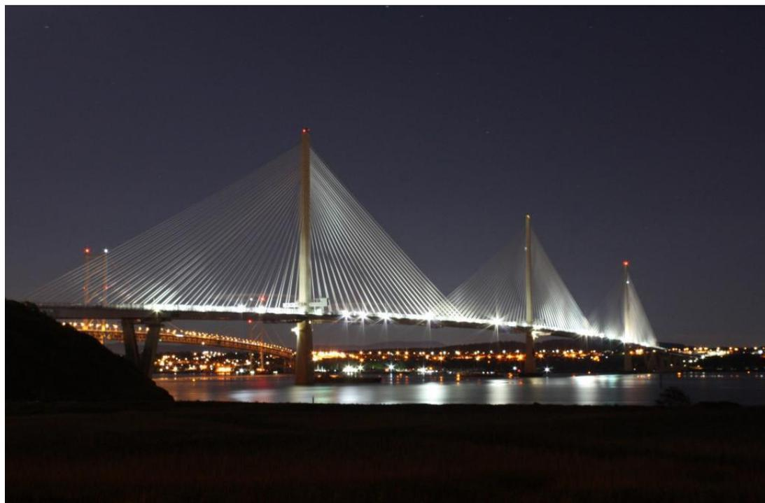
2,610 custom-made Deckedge LED luminaires turn the functional 3m high acrylic windshield into an aesthetic feature.
