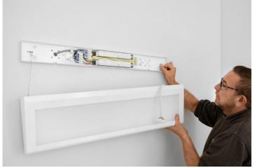
A 5-pin plug-and-play terminal is provided for easy wiring of both the downlight and uplight
