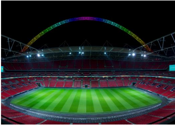
Thorn replaced the stadium's iconic arch lighting with a custom LED lighting system designed for full colour as well as special moving light effects.
