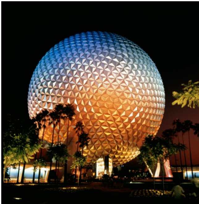
The 49 m diameter globe named "Spaceship Earth" which is the symbol of EPCOT Centre in Florida, was floodlit by Thorn CSI lamps in 1983
