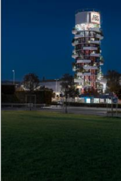
The imposing water tower at the entrance of the ABS site is showcased by SUPERSYSTEM outdoor from Zumtobel and Contrast LED from Thorn.
