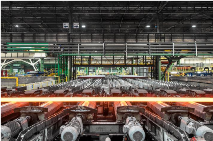
CRAFT from Zumtobel provides both uniform hall lighting and efficient illumination of the high-rack storage sections.
