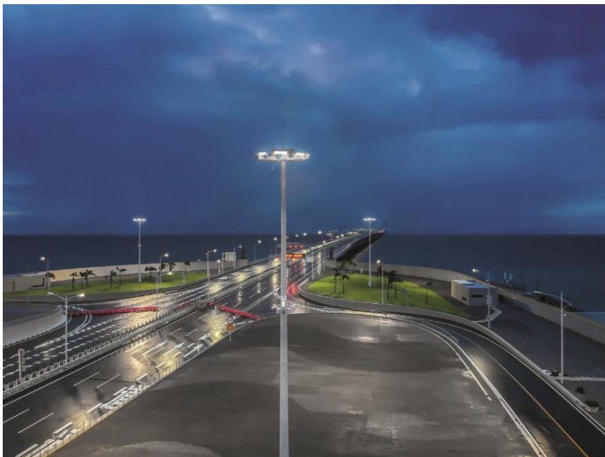
Thorn provided 120 Champion Pro LED 132 high-power floodlights, mounted on 12 high masts.
