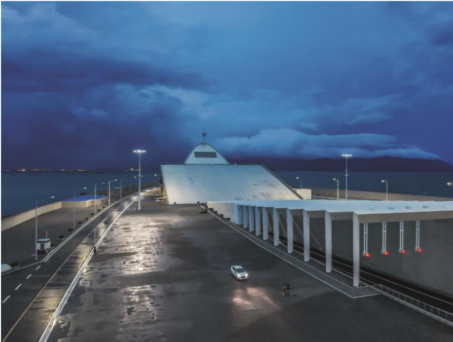
Thorn was able to meet the extremely high construction standards and rigorous technical criteria.
