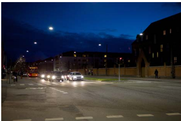
Most street lanterns in Copenhagen are catenary mounted above the road, depending on the size of the road in one or two rows.
